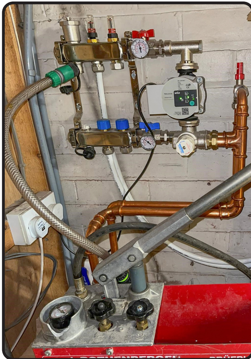
Figure 3 - using a test pump to pressurise the system to 5 bar
